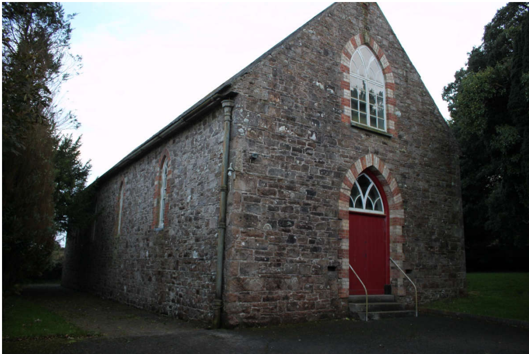
Church on Chapel Hill – one Soprano pipistrelle emerged from under the slates at dusk
