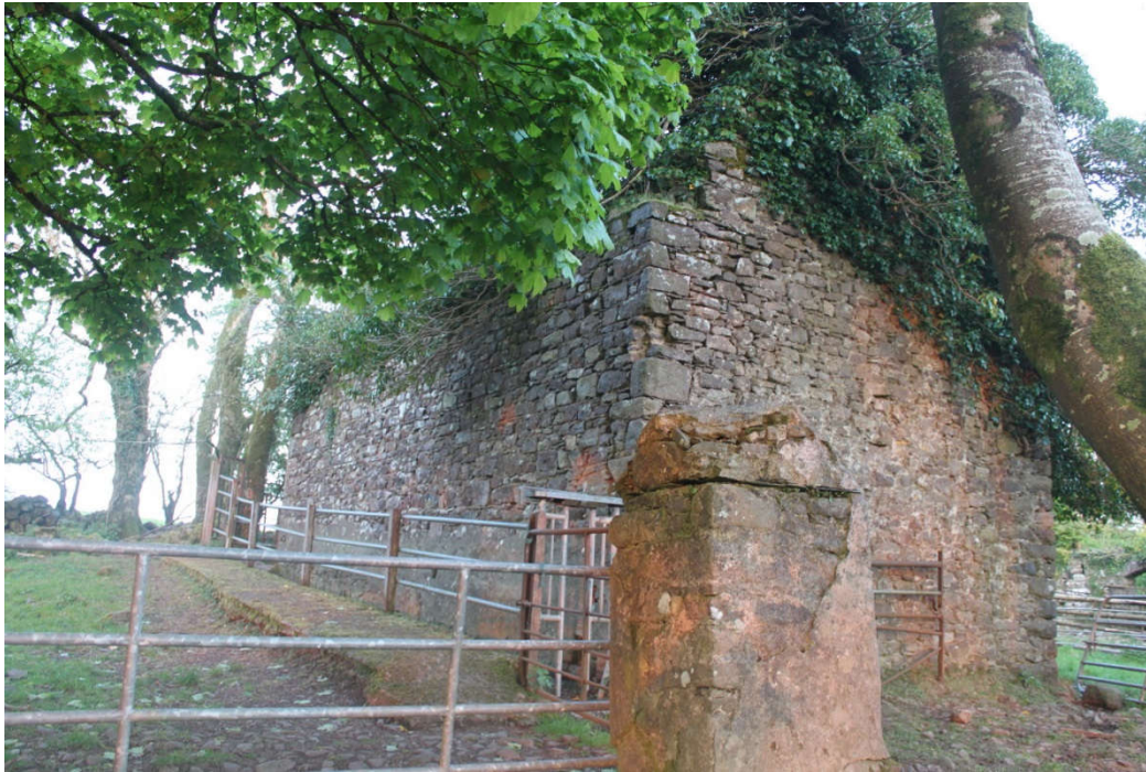
Photo 22 - Eddie Dempsey's stone farm buildings (Grid Ref S58279 32302)
