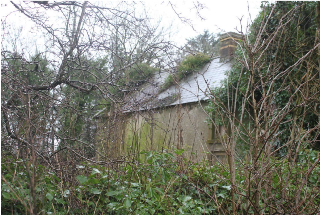
Photo 19 – Two storey farmhouse in ruins at Castlebanny townland c1.7km west of site boundary.
