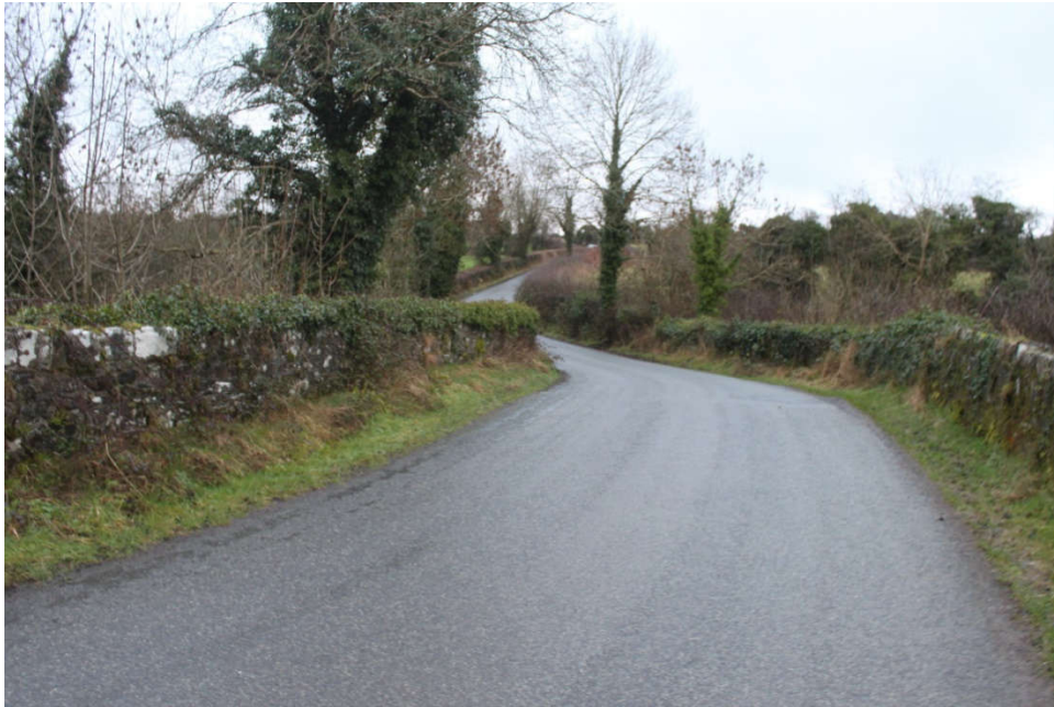
Photo 17 – Ballyconway Bridge - masonry bridge over tributary of Little Arrigle River situated c1.7km north of proposed site
