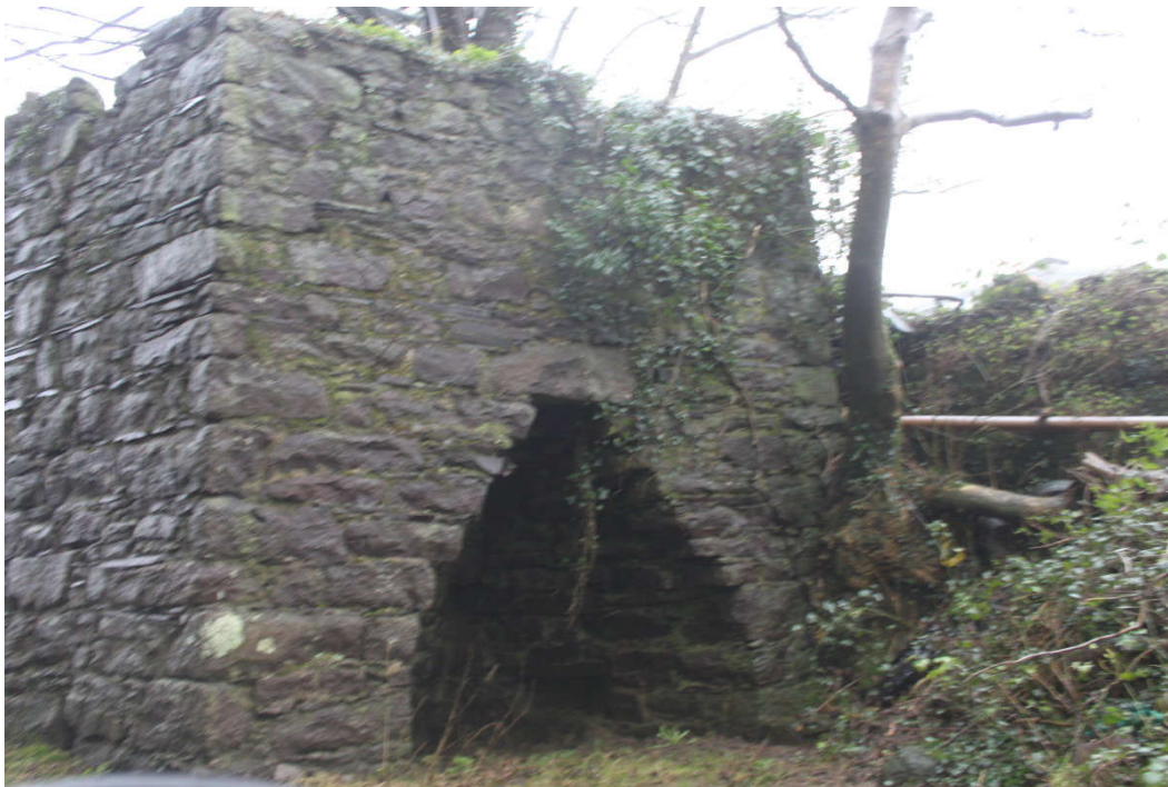
Photo 20 – Stone structure (lime kiln) at Ballytarsna townland c. 2km west of site boundary
