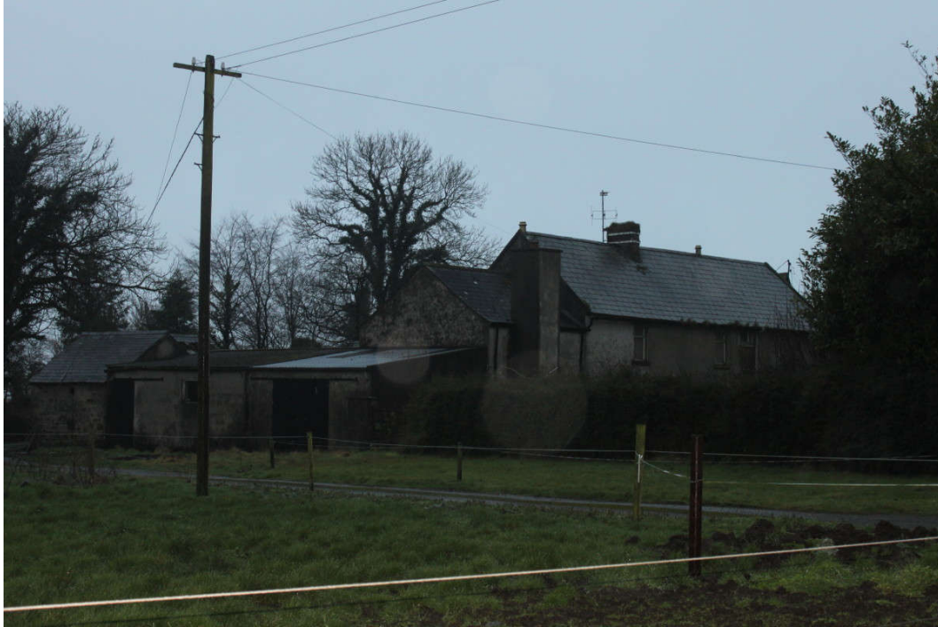
Photo 9 – Disused farmhouse and outbuildings at Castlebanny townland on entrance lane to the proposed Springfield Wind Farm
