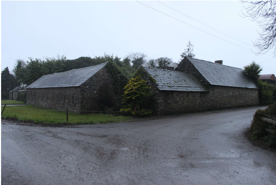
Photo 7 – Group of old stone farm buildings with natural slate roofs at Castlebanny townland on entrance lane to the proposed Springfield Wind Farm. These buildings lie c.1.2 km to west of site boundary
