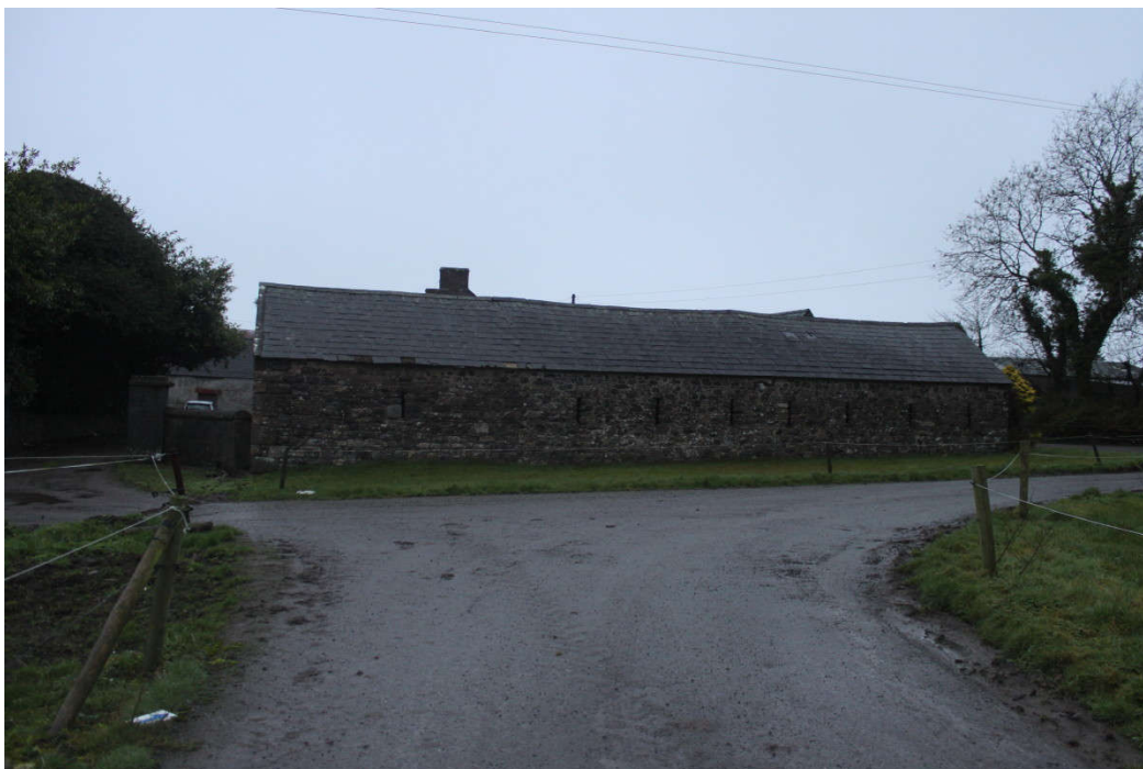
Photo 8 – Long stone farm building with natural slate roof at Castlebanny townland (as above)
