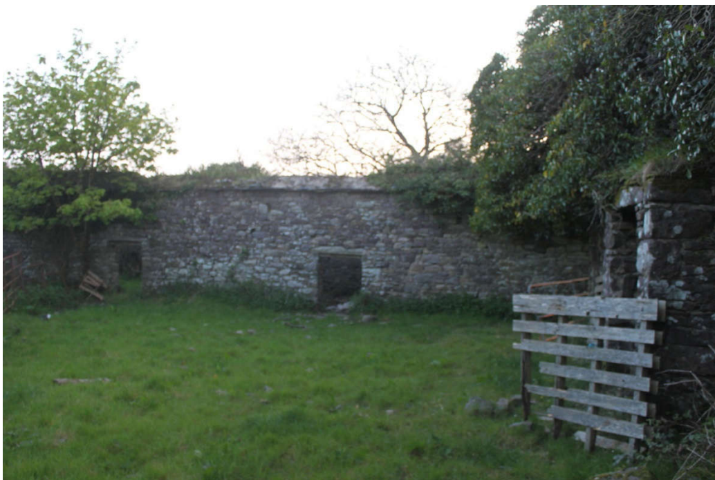
Photo 25 - Eddie Dempsey's stone farm buildings (Grid Ref S58279 32302)
