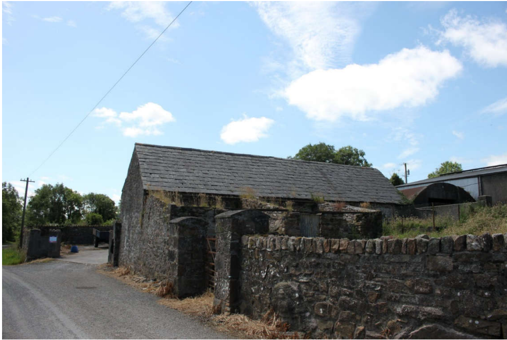
Photo 40 - Shed in Coolroebeeg Townland (Grid ref S593 348). A single Brown long-eared bat and a single Soprano pipistrelle entered the roof space at dawn
