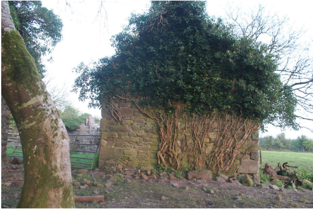
Photo 24 - Eddie Dempsey's stone farm buildings (Grid Ref S58279 32302)
