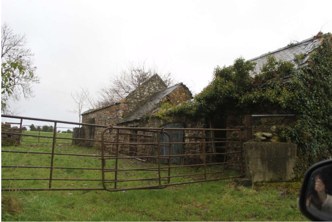
Photo 15 – Dilapidated Farm buildings on Chapel road, Powerswood within proposed area of site
